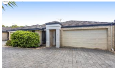
Unit 5, 14 Binnar Ct, Erskine
