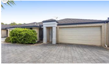
Unit 5, 14 Binnar Ct, Erskine
